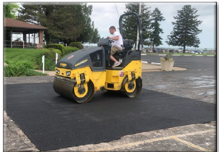
A steamroller smooths out our new parking lot.
